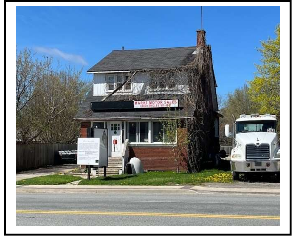
View to west from Highway 27 toward 12966 Highway 27.
