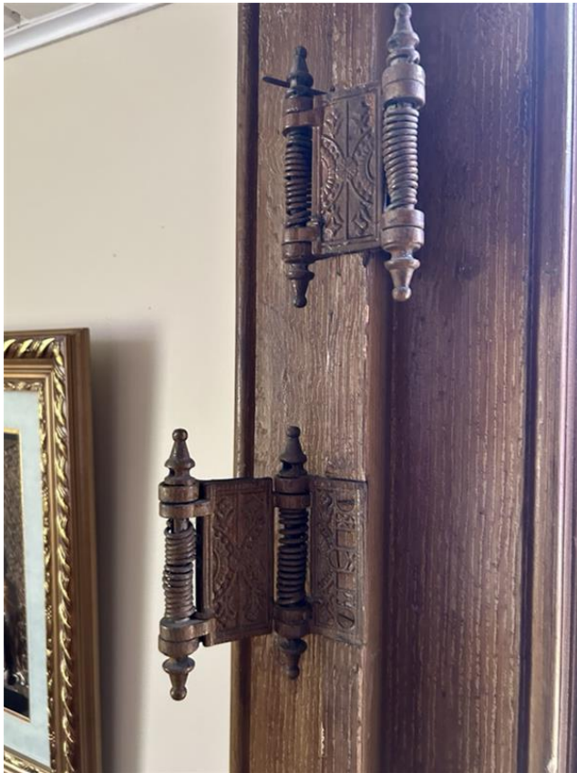
Figure 8. Original decorative door hinges. (King Township Staff, 2025).
