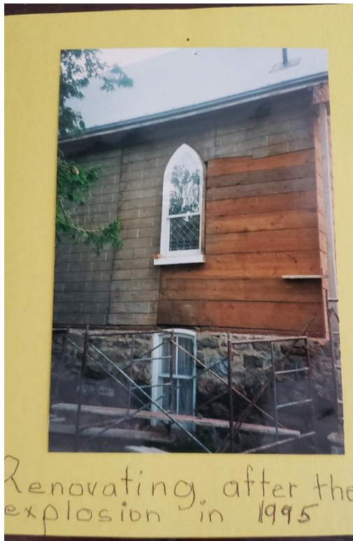
Figure 12. Archival photograph of subject structure with brick-cladding removed. Note the distinct former window cutout, which has neo-classical features. Also note the wooden boards made to resemble etched stone blocks. (King Township Archives, n.d.).
