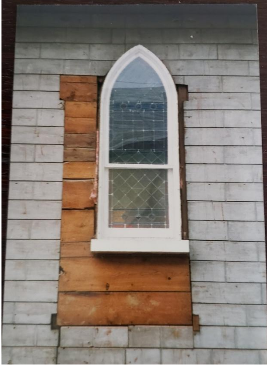
Figure 13. Archival photograph of subject structure with brick-cladding removed. Note the distinct former window cutout, which has neo-classical features. Also note the wooden boards made to resemble etched stone blocks. (King Township Archives, n.d.).
