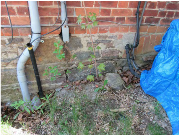
Figure 34: Foundation at north wall
