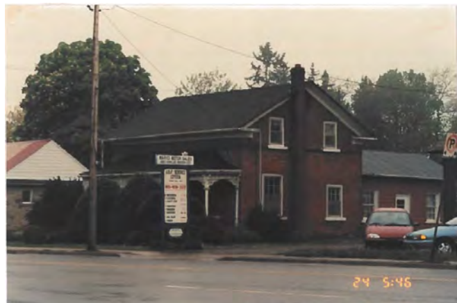
Figure 27: Northeast Elevation of the subject property c.2000. The rear addition is extant at this time and visible at the right (Township of King Records)
