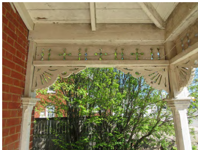
Figure 50: Woodwork detail at north end of verandah
