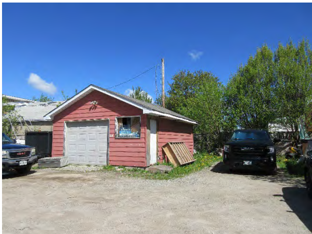
Figure 14: Garage at rear of property with shed to its left
