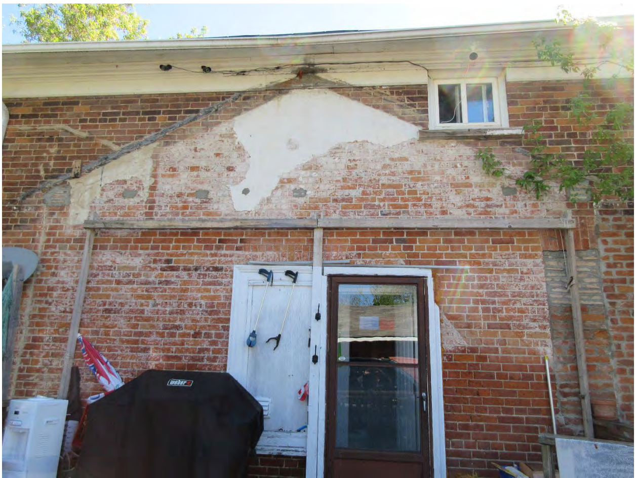
Figure 31: Rear (west) elevation where there is evidence of the former tail having been removed
