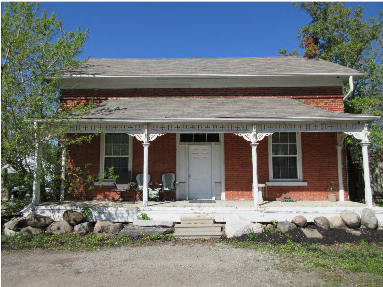
Figure 30: Front (east) Elevation
