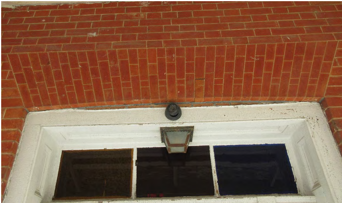
Figure 43: Brick segmental arch above front door transom with contemporary light fixture and security camera
