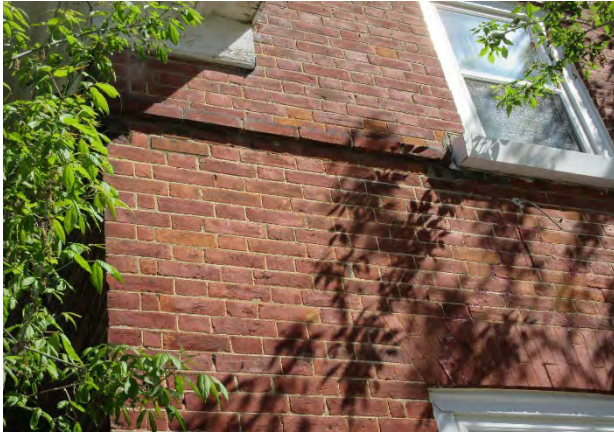
Figure 32: Masonry laid in Flemish bond and brick string course aligning with underside of 2 nd floor window sills
