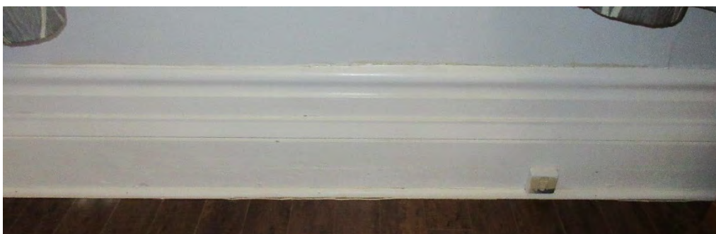
Figure 52: Tall floorboard on main floor
