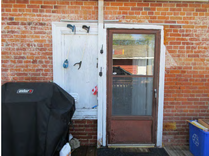
Figure 44: Rear entrance door with wood cutout.
