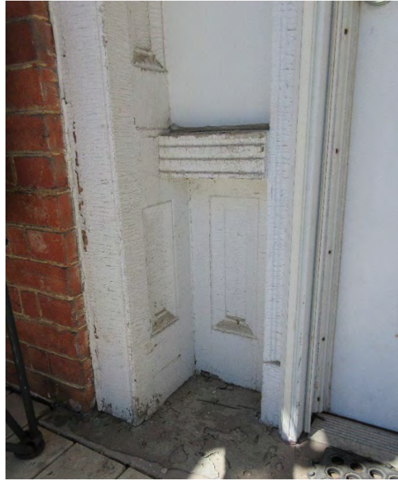
Figure 42: Wood panelled detailing below sidelights
