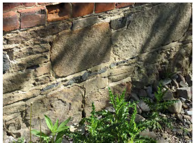
Figure 35: Foundation at south wall
