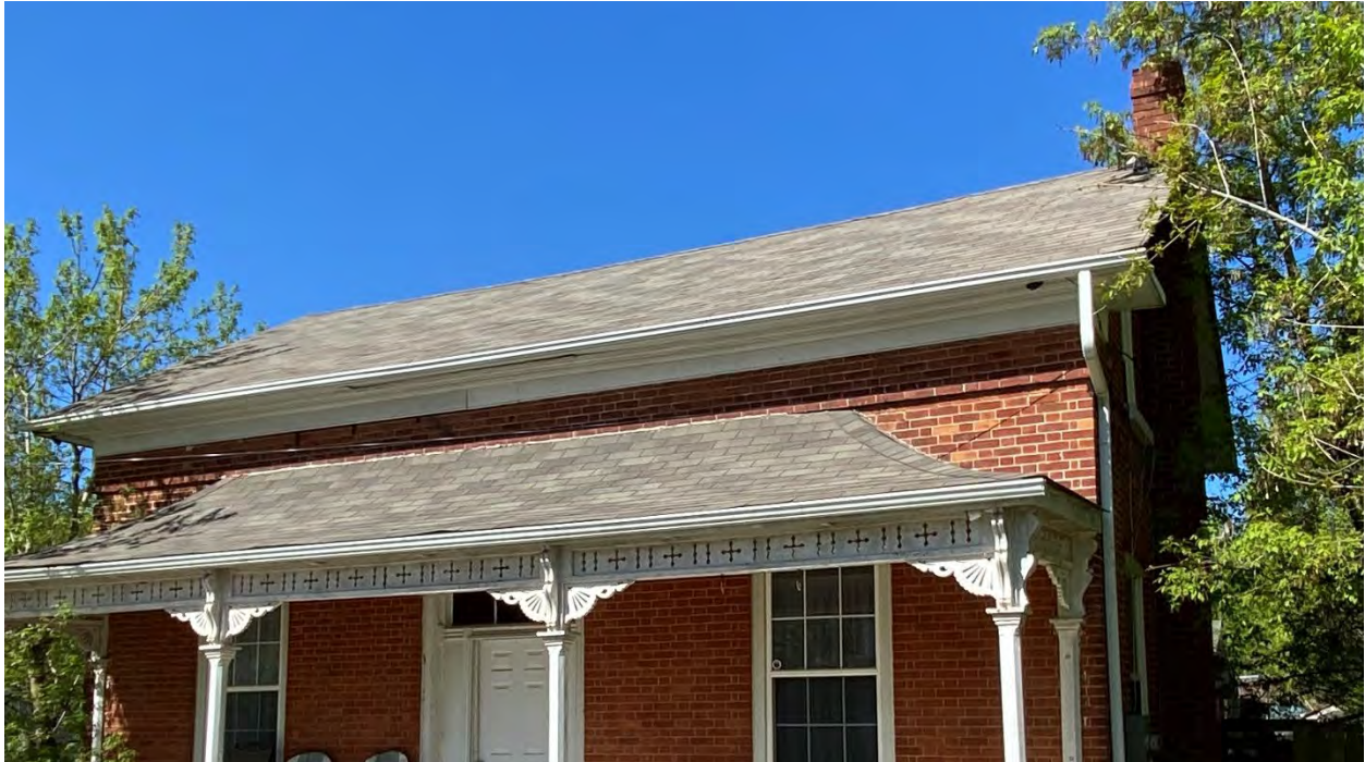
Figure 36: Asphalt shingle roof
