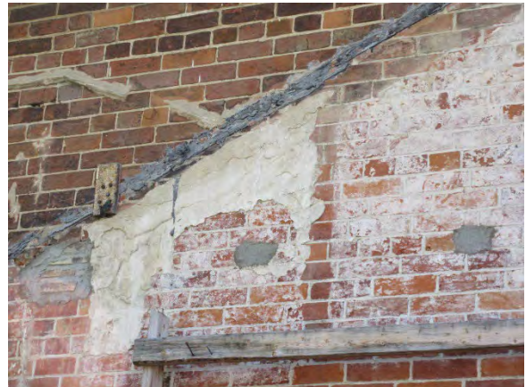
Figure 33: Masonry within area of former rear addition.
