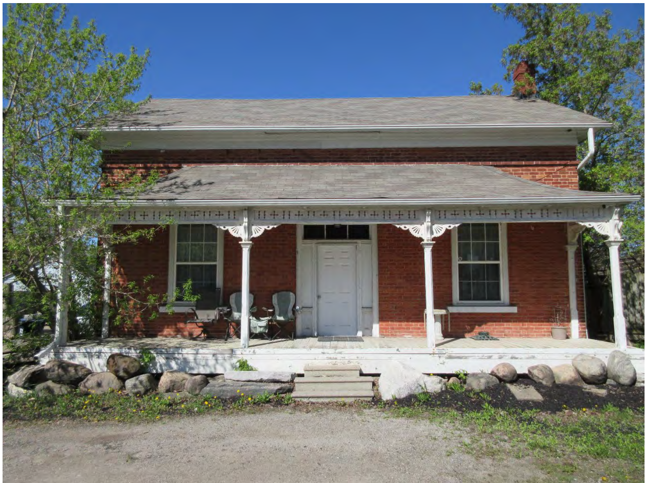
Figure 5: East (Front) elevation of the subject property.
