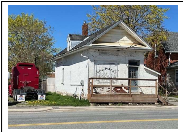
View to west from Highway 27 toward 12972 Highway 27.
