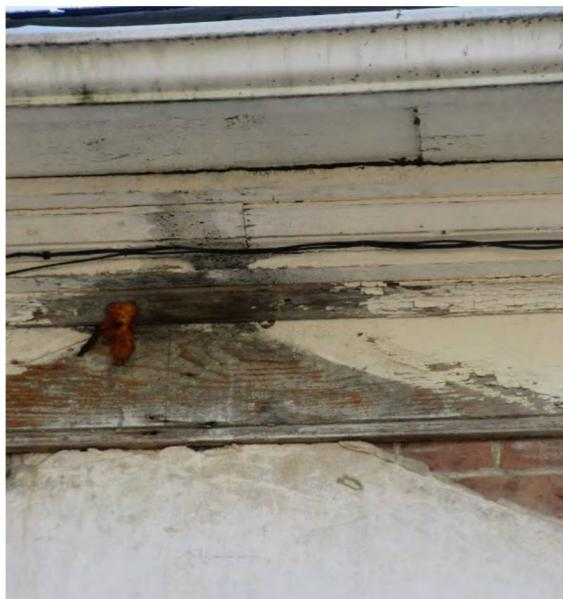
Figure 47: Bare wood where former tail was removed
