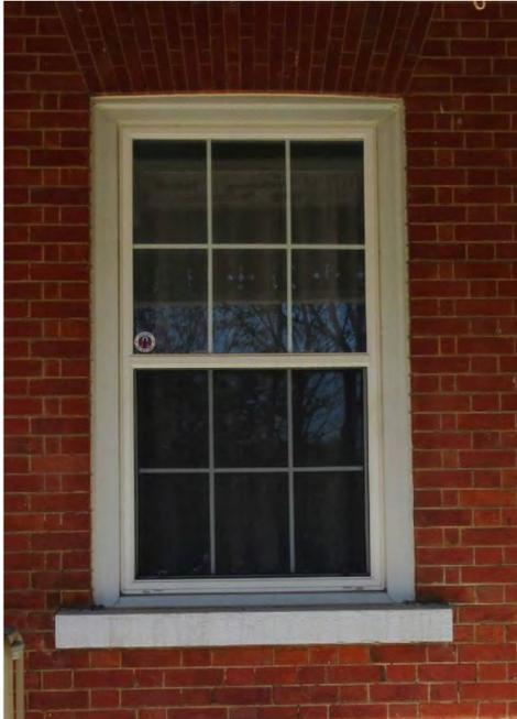
Figure 38: Front window with segmental arch
