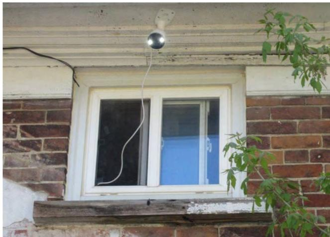
Figure 40: Rear upper vinyl window with wood sill
