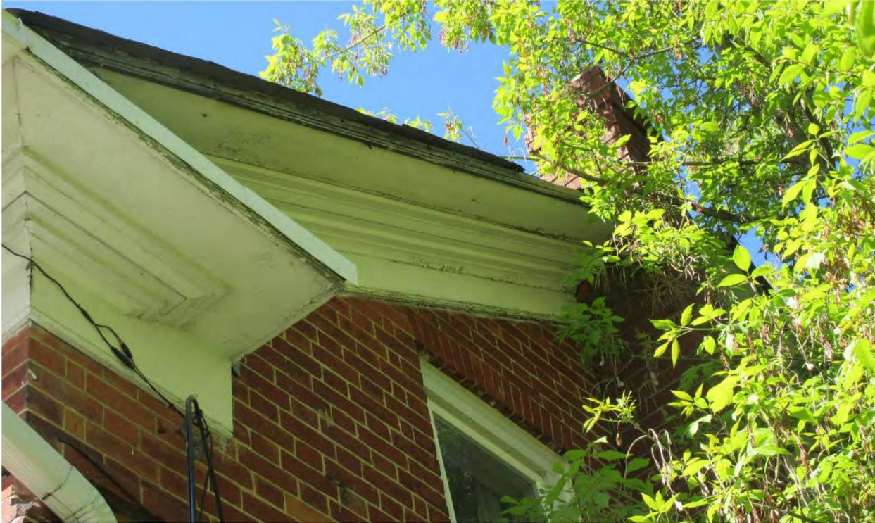
Figure 46: Fascia and soffits at roofline along north with wood return at far left
