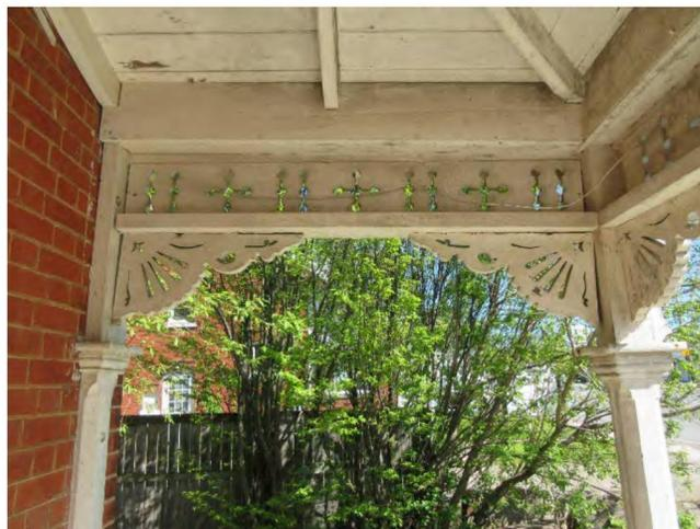
**Figure 50:** Woodwork detail at north end of verandah
