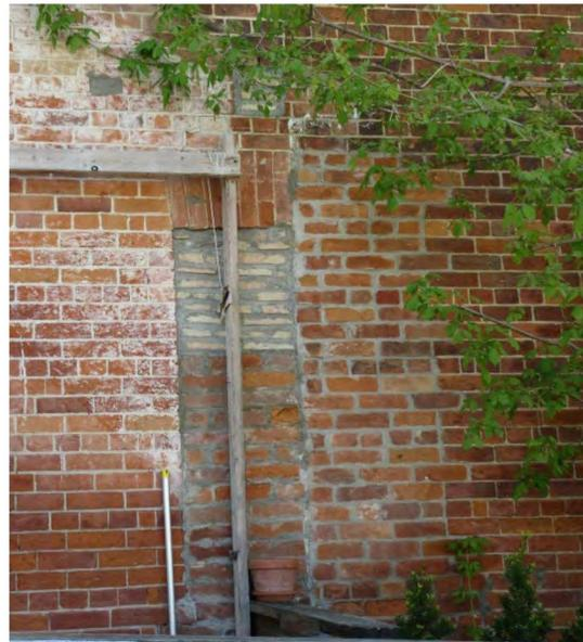
**Figure 45:** Former masonry opening with brick infill
