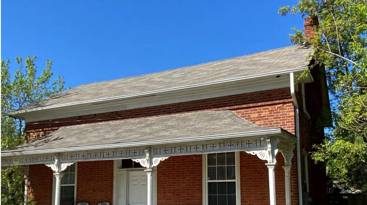
**Figure 36:** Asphalt shingle roof
