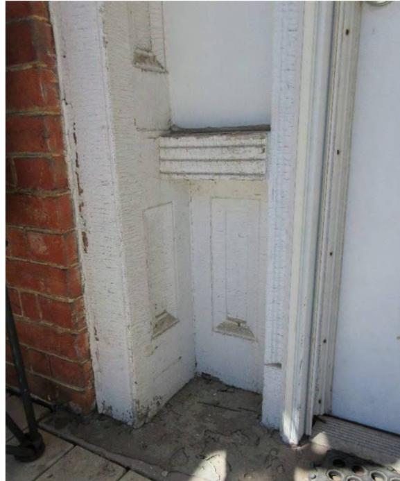
Figure 42: Wood panelled detailing below sidelights
