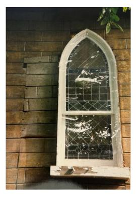
Figure 14. Archival Photograph of subject strucutre with brick-cladding removed. Note the distinct former window cutout, which has neo-classical features. Also note the wooden boards made to resemble etched stone blocks. (King Township Archives, n.d.).
