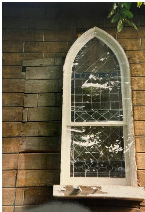
**Figure 14.** Archival Photograph of subject structure with brick-cladding removed. Note the distinct former window cutout, which has neo-classical features. Also note the wooden boards made to resemble etched stone blocks. (King Township Archives, n.d.).
