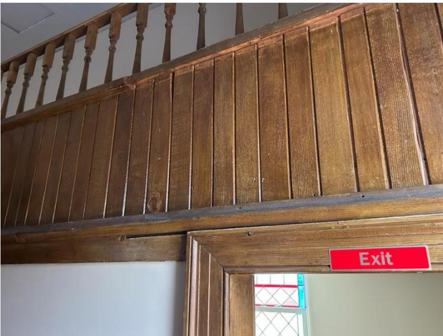
**Figure 10.** Original wainscoting with painted-on wooden grain. (King Township Staff, 2025).
