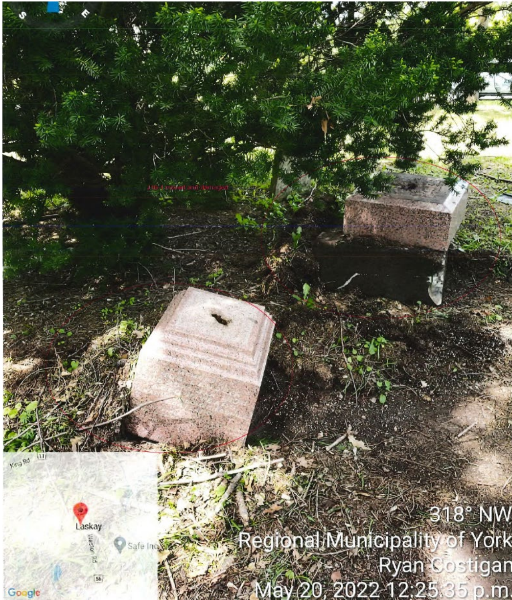
Figure 36: J16-1 disassembled, with top stone at left and bottom and middle stones at right (Ryan Costigan 2022).
