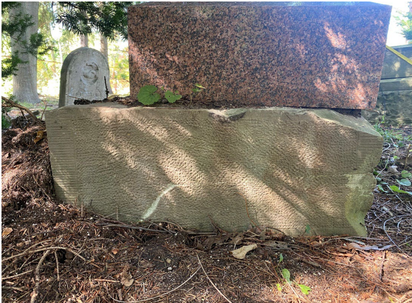
Figure 39: J16-1 scratches on bottom stone from machinery, looking east (A.S.I., 2023).
