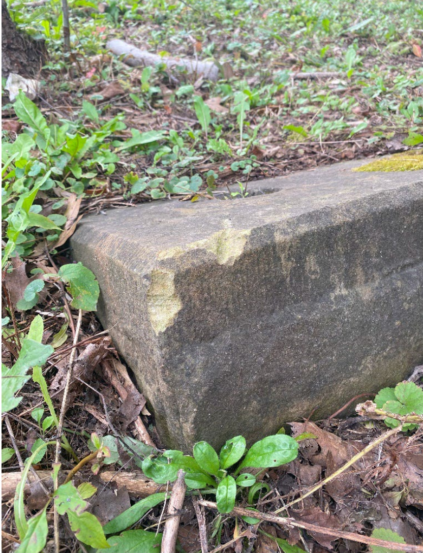
Figure 58: J20 – Gouges from machinery (A.S.I., 2023).
