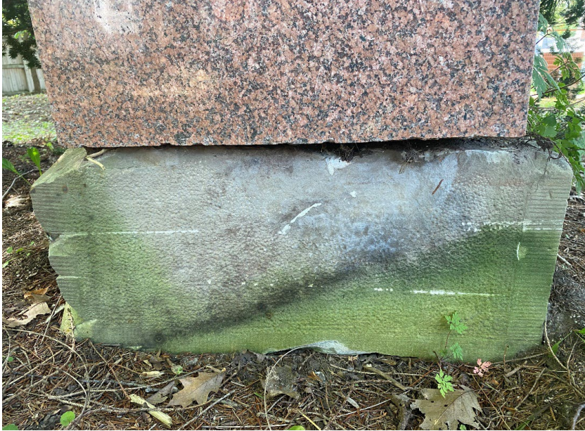
Figure 40: J16-1 scratches on bottom stone from machinery, looking south (A.S.I., 2023).
