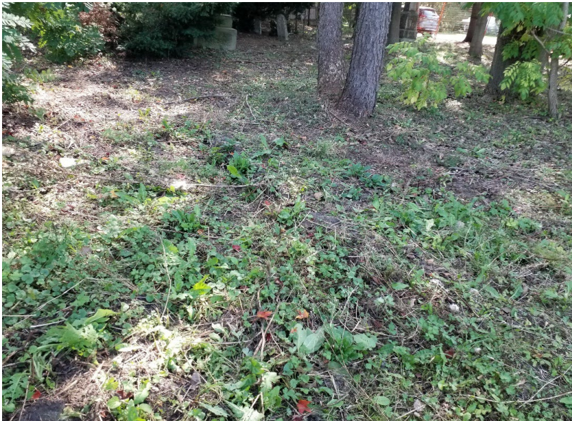
Figure 18: Ruts left by construction equipment in May 2022, near the northern end of the property (A.S.I. 2023).
