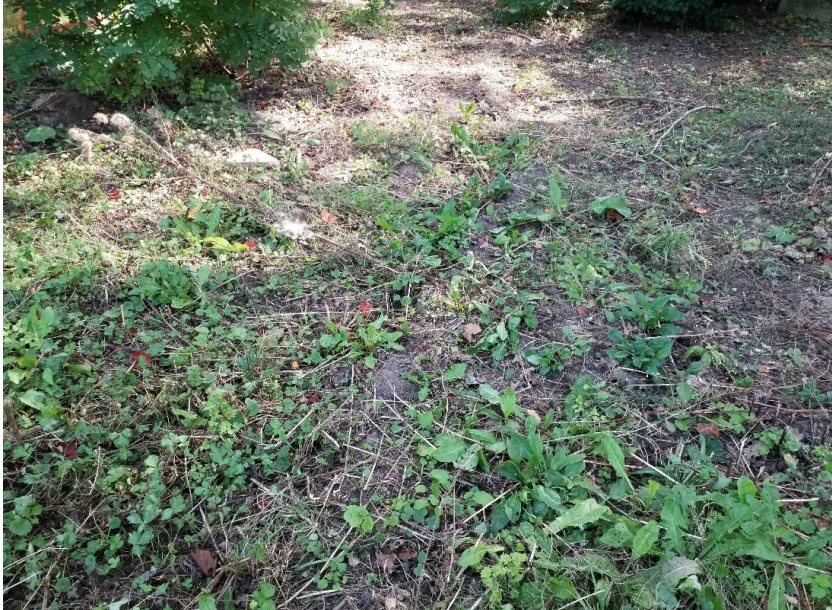
Figure 17: Ruts left by construction equipment in May 2022, near the northern end of the property as documented in September 2023.
