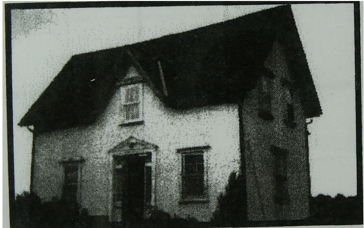
Figure 1: Tollgate Keepers House, located at 650 Toll Road
