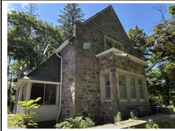
Photo #5: Photo taken facing northwest. Staff note the screened porch as not being original to the structure.
