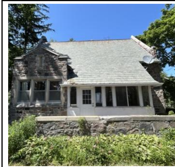
Photo #1: South facing elevation of gatehouse. Staff note the screened front porch, and windows are not original to the structure.
