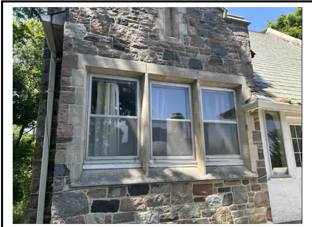
Photo #7: Windows on south facing elevation of gatehouse. Staff note the existing window openings will not be altered, and the proposed windows will be retrofitted into the existing openings.
