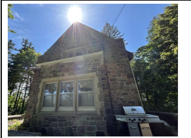
Photo #4: East facing elevation of gatehouse.
