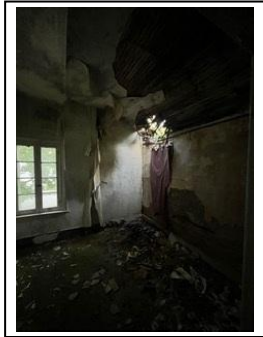
Photo #9: Images of the interior provided by the applicant. Staff did not enter the structure due to safety concerns.
