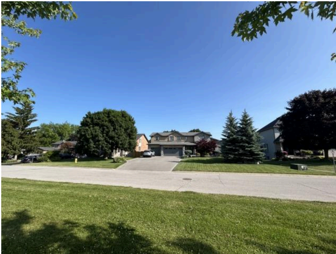
Pic 12: In Park standing in front of baseball diamond 1 looking south on Janet. These 2 stories are no more than 9m and have lots of space around them.
