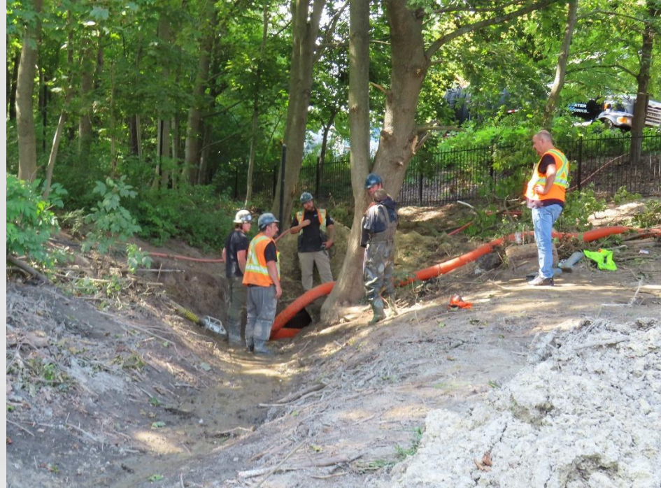
King's contractor cleaning drainage pipe on my property to be ready to receive water from hundreds of meters of drainage from Snowberry & Kingscross
