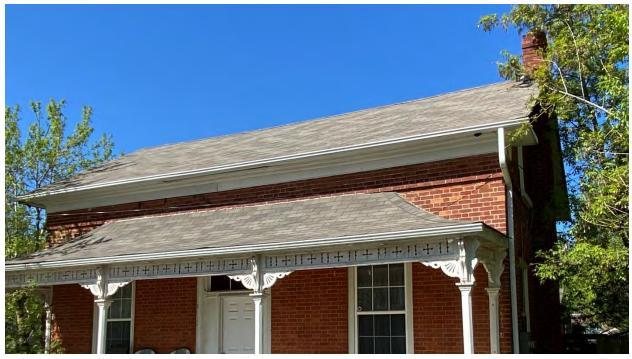
Figure 36: Ashphlat shingle roof
