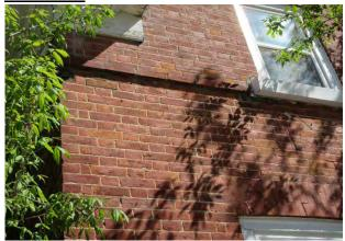
**Figure 32**: Masonry laid in Flemish bond and brick string course aligning with underside of 2<sup>nd</sup> floor window sills
