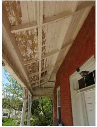
Figure 49: Underside of porch roof with peeling paint on wood
