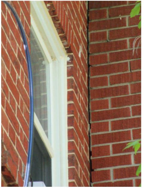
Figure 37: Close up of chimney where older brick is visble at left in contrast to new brick of the chimney at right
