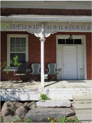
Figure 48: Porch with decorative wood trimwork and columns
