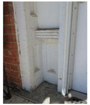
Figure 42: Wood panelled detailing below sidelights
